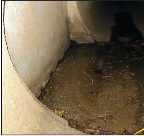
Figure 20. Accumulation of sediment in the junction of a manhole with the storm-sewer conveyance system.
